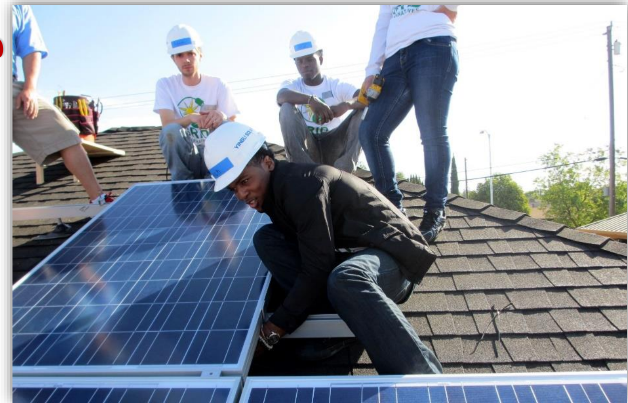
On the Job Training
